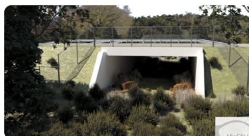
The tunnel allows animals to go under the highway to cross it, preventing them from being run over
